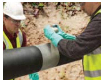
Tightly wrap repair area
