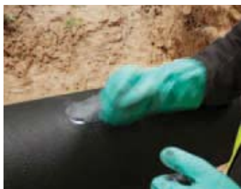
Mix and apply epoxy putty
