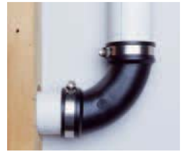
The extra length of the Qwik Ell completes the repair
